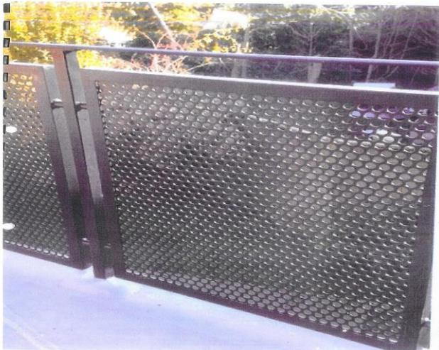
The perforated panel will be powder coated prior to installation, largely removing the need for future decoration
